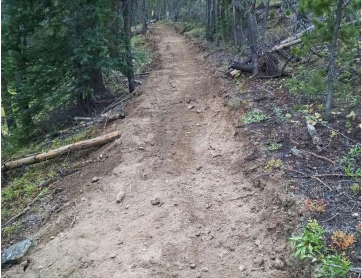
ATV trail constructed by District Staff using a mini-excavator
