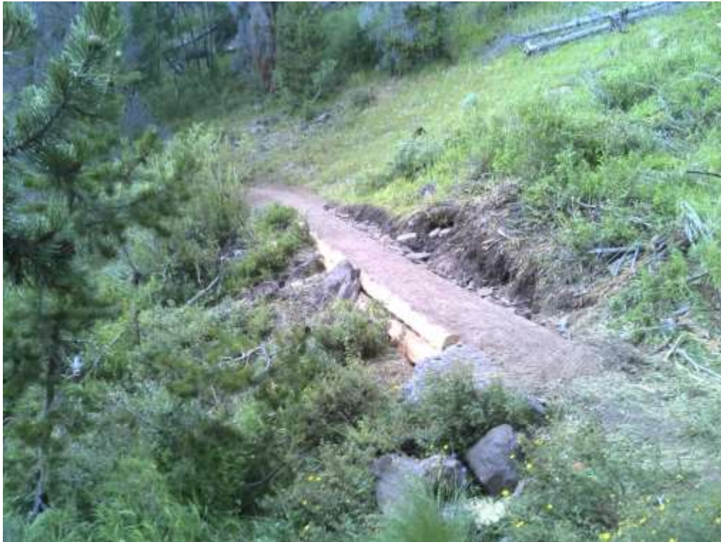
Turnpike constructed by the Colorado Statewide OHV Crew.
